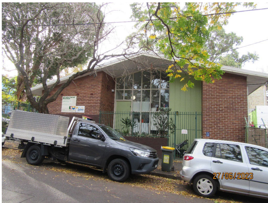
15 Eastern elevation of the kindergarten facing Phelps Street, showing the principal entry and porch.
