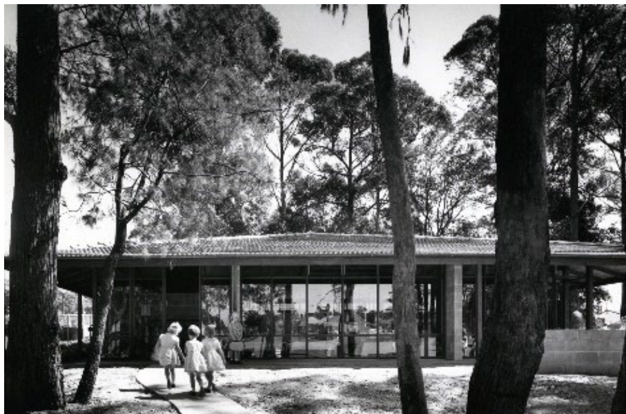
35 The kindergarten at St Ives designed by Collard Clarke & Jackson.
